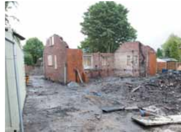
The demolition of the old property is nearly complete
